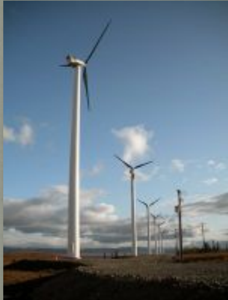
Unalakleet wind turbines
