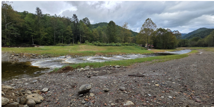
Eastern Band of Cherokee Indians - Dam Removal Project
